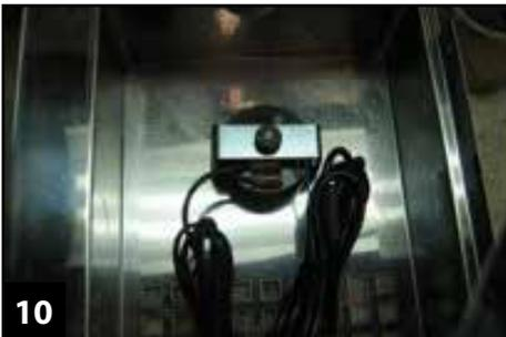
**STEP 15** - Remove thumb nut and bracket on back side of thermometer (See image 10)
