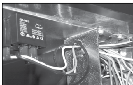
7 - Routing relay wires
