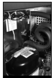
Placement of Relay (above compressor)
