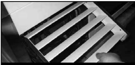
2 - Louvered grill hinges out then unhooks for removal
