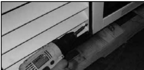
1 - Removing two (2) lower screws
