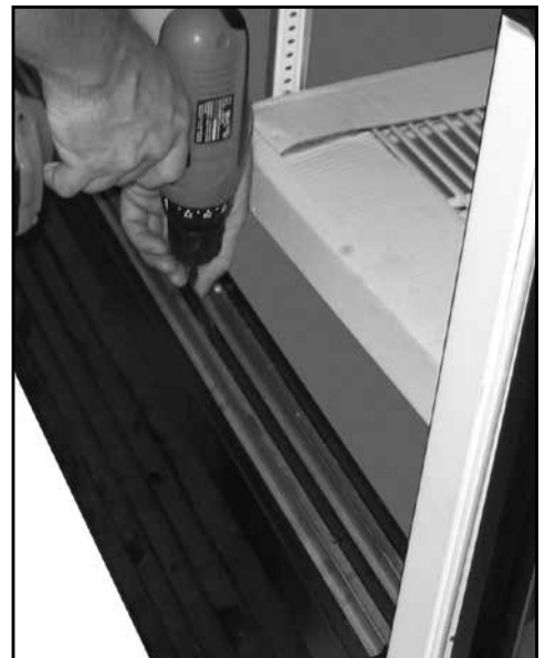
3 - Removing old V-Track
