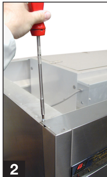
2 Three Door Freezer unit (Rainshield Removal/top screws)
