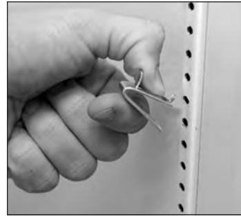
Fig. 1. Installing top tab of shelf clip.
