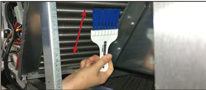
Fig. 3. Never brush across the coil fins.
