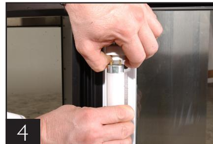
The lamp holders are spring activated. Pull the top lamp holder up and push the bulb down at the same time. This will leave enough clearance to remove the bulb.
