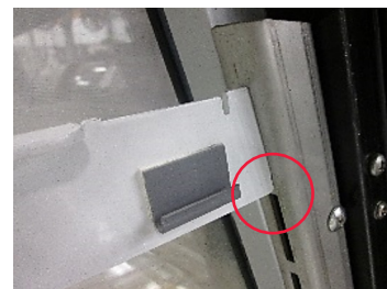
Bottom notch installed (no gap)
