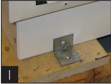
Removing skid from bottom of cabinet.
