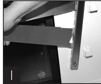
1 Install shelf supports. teeth end into stainless pilasters.
