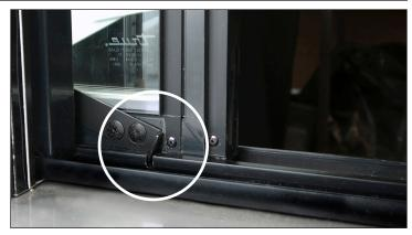
Fig. 1. Door latch is in the open position (engaged with notch).
