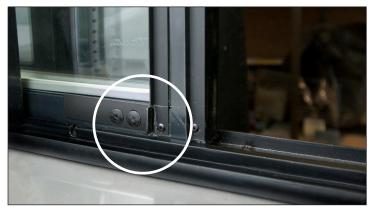
Fig. 2. Door latch is in the closed position (disengaged from notch).
