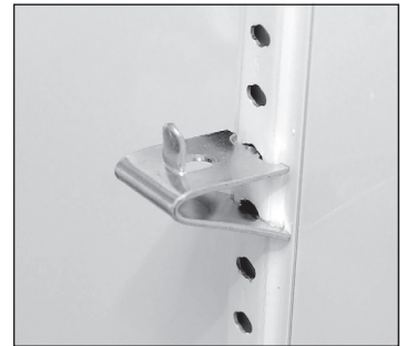
Fig. 4. Installed shelf clip.
