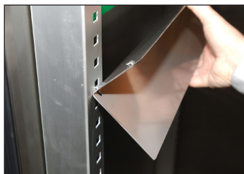
Fig. 7c. Installing kit #3 universal tray sides.
