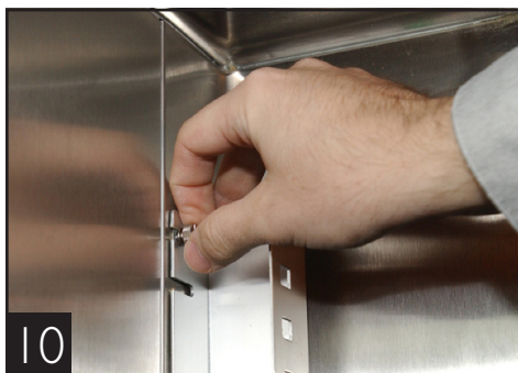
Pilaster installation (side wall of cabinet)
